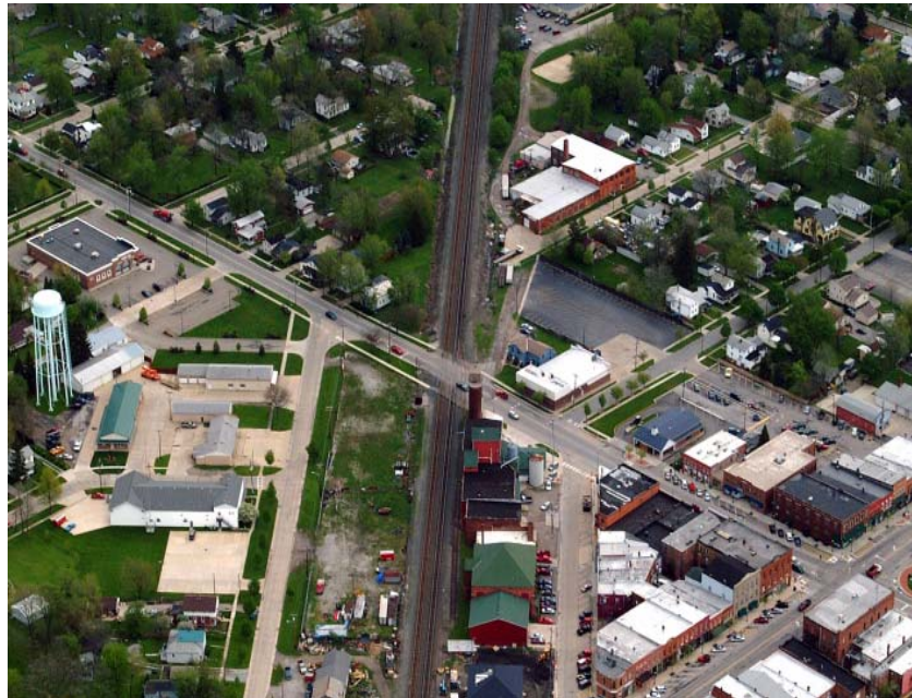
Figure 1: Existing alignment looking northeast
