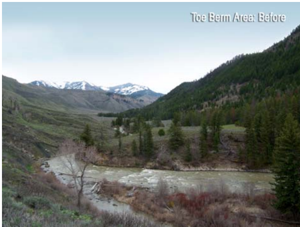
Figure 4: Toe Berm Area – Before
